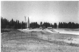
View of Atlas-E ICBM Serial #58-7135 (19E) raised and GOXing ("breathing") at LC 567-9, Reardan/Long Lake, WA., 22 July 1961. (Convair/General Dynamics Photo) Image courtesy of www. Silsoworld.com
