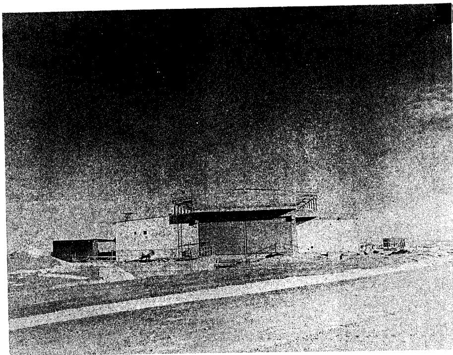
Date: Jan 19, 1960, DA-5498, F.E. Warren AFB Launch Facil Squad II Site C, Launcher #3, view looking east shows flame pit, GOX, and Nitrogen Areas. Tanks and skids have not been placed.
